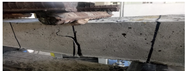
5(a) shear crack in beam specimen pt: 3.92(a/d=1.25)
